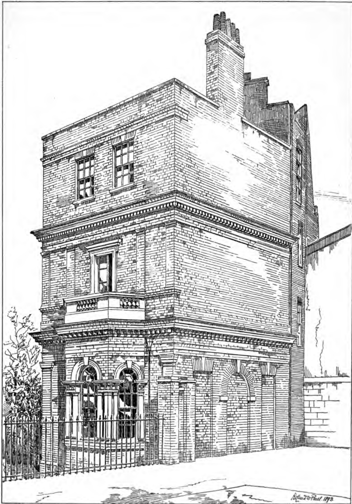
THE GARDEN HOUSE, CLEMENT'S INN, FROM N W
